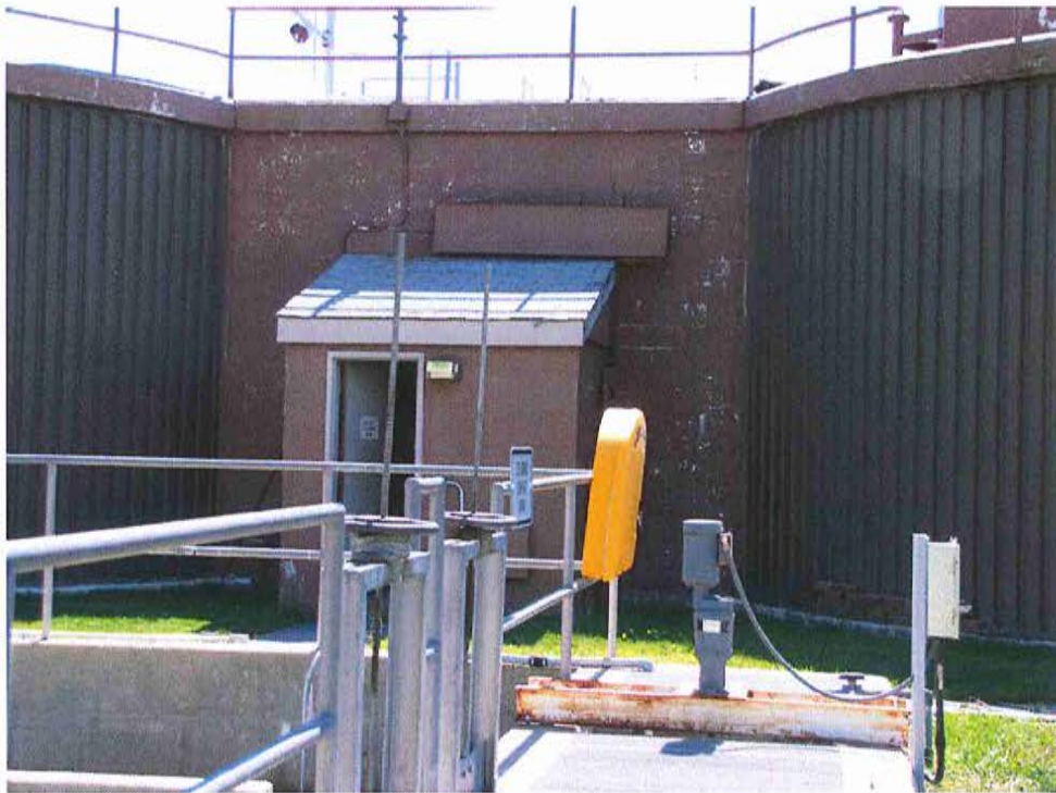
Photo 89: Sludge Storage Tanks - View of north connector wall with failed paint on masonry block.
