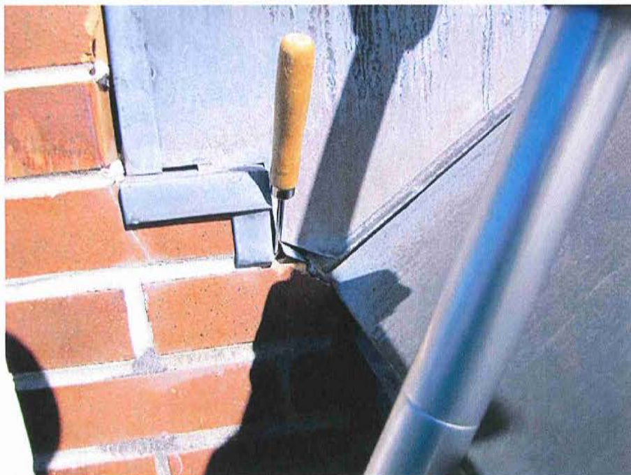
Photo 35: Lab/Admin - Roof to wall flashing conditions at the south face of the wall end shown in photo 29. Note water can enter brick veneer cavity where the ice pick is stuck down into brick wall. Note ragged edge of brick ends and no sealant at vertical joint with wall flashing. Open joints between flashing and brick permit water entry into the wall.
