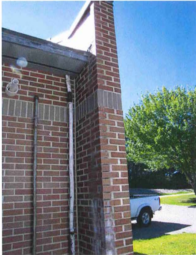
Photo 40: Lab/Admin - North end of west wall. Note shadow below parapet wall cap flashing. Wall flashing has pushed inwards. See close up photo #41.
