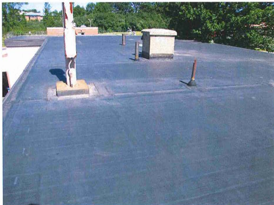
Photo 62: Control Building - View of roof membrane looking north. Trees should be pruned back to prevent branches from sitting on membrane. Masonry block chimney needs re-pointing. Roof membrane is in good condition.
