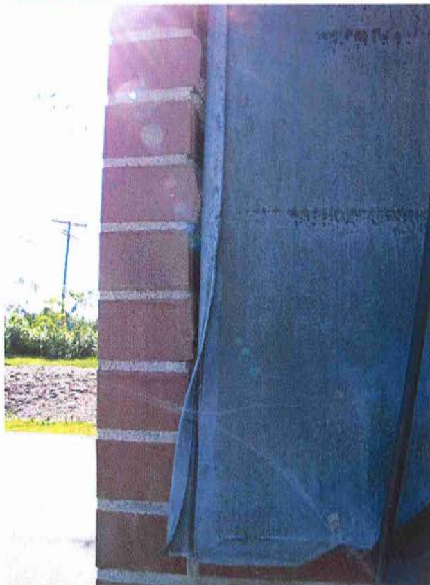
Photo 17: Lab/Admin - SE corner showing flashing termination seam being unfolded and lack of any sealant between metal flashing and brick veneer. Note jagged ends of brick in alternate courses, because bricks were not saw cut.
