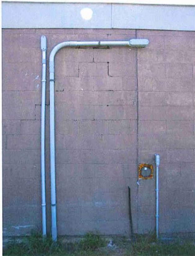
Photo 68: Intermediate Pump Station - View of repaired NW corner. Roof slopes down from right to left, permitting water to run down the face of the north (left) CMU wall.
