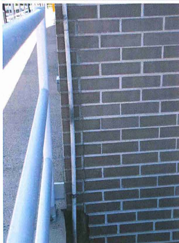
Photo 103: Blower Building - Close up of NE corner of building at 2 nd floor level, showing crack extending up 9 brick courses above walkway of SBR tank. A control joint should be cut in place at this location.
