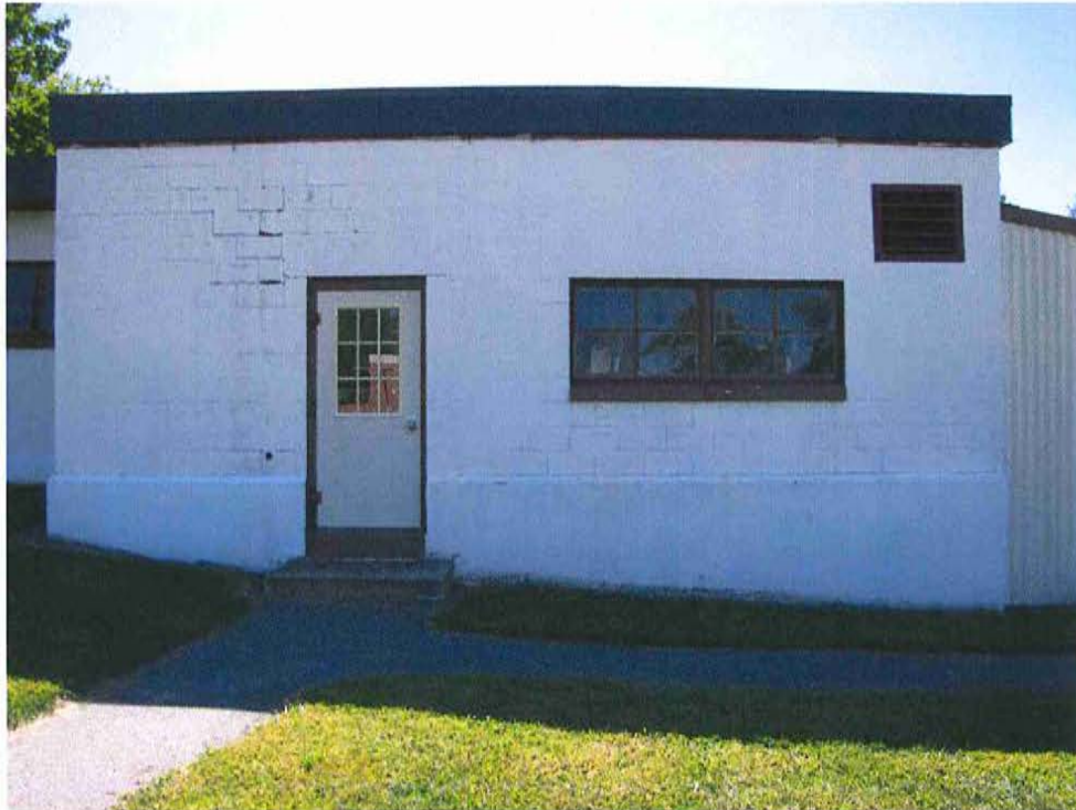
Photo 57: Control Building - North wall of grit room addition showing cracked masonry below the large window and above the door.
