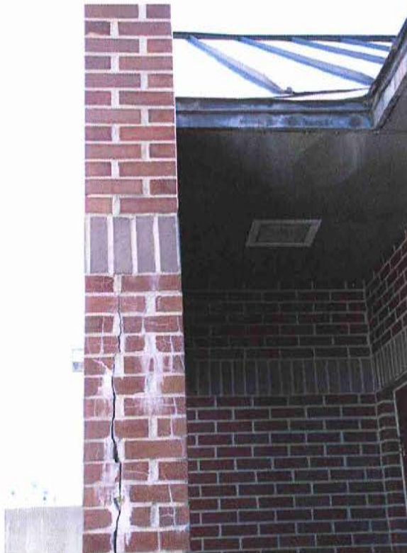
Photo 29: Lab/Admin - Closeup of NW corner of roof above main entry into building. Note severe crack in brick pilaster end.
