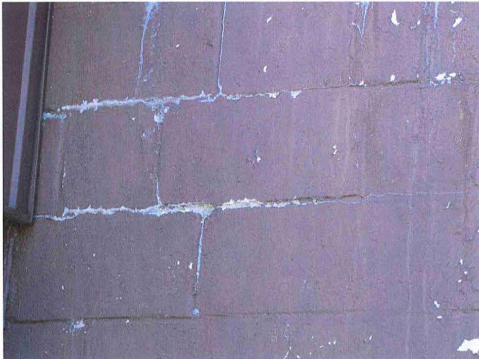
Photo 92: Sludge Storage Tanks - Close up of photo 89, to the right side of small room with shed roof, showing mortar joint cracking and deterioration.
