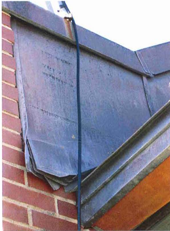
Photo 11: Lab/Admin - SE corner showing flashing at wall at bottom edge seam being unfolded by sliding snow and ice.
