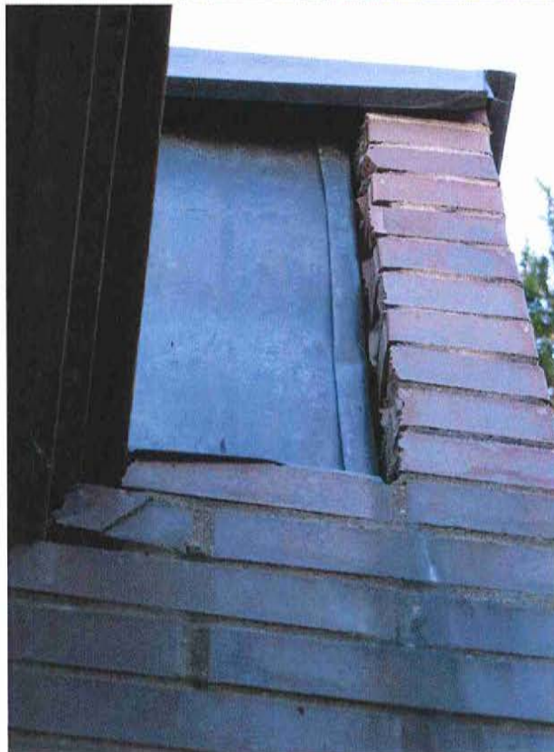
Photo 41: Lab/Admin - Close up of metal flashing conditions from photo 40. There is insufficient backup material behind wall flashing to hold it in its proper location. Brick ends are ragged, preventing sealing to the folded flashing seam. There is no backer rod or sealant at the flashing to brick joint to prevent water infiltration. Sliding snow can easily get into this joint.
