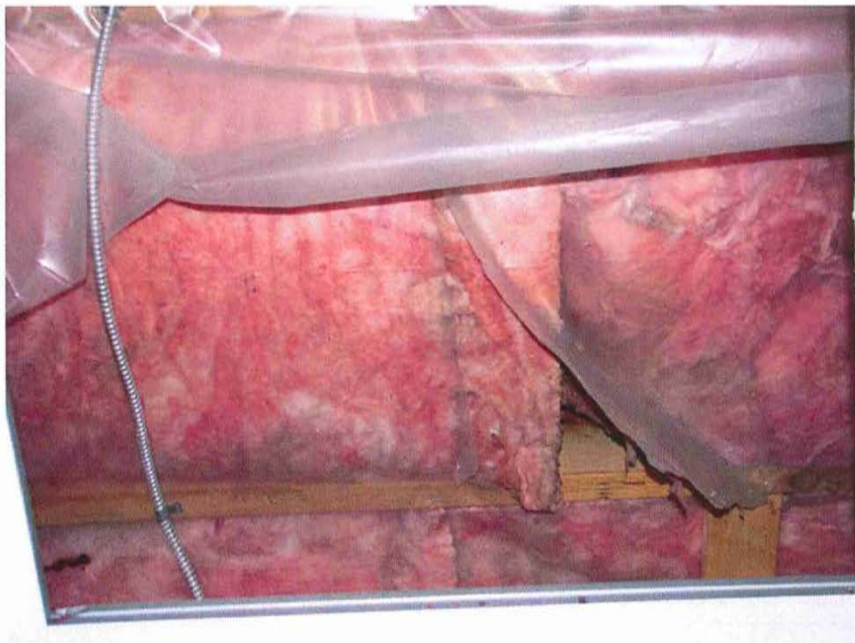
Photo 43: Lab/Admin - Vapor barrier and insulation conditions above women's room, permitting heat and moisture to escape into the attic space.
