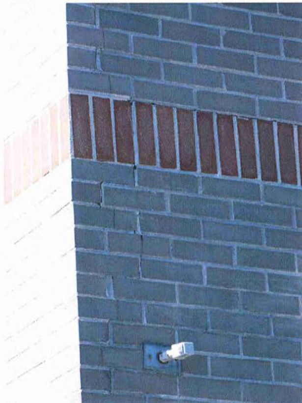
Photo 100: Blower Building - Close up of photo 99 showing cracked brick veneer. A control joint is needed at this location.
