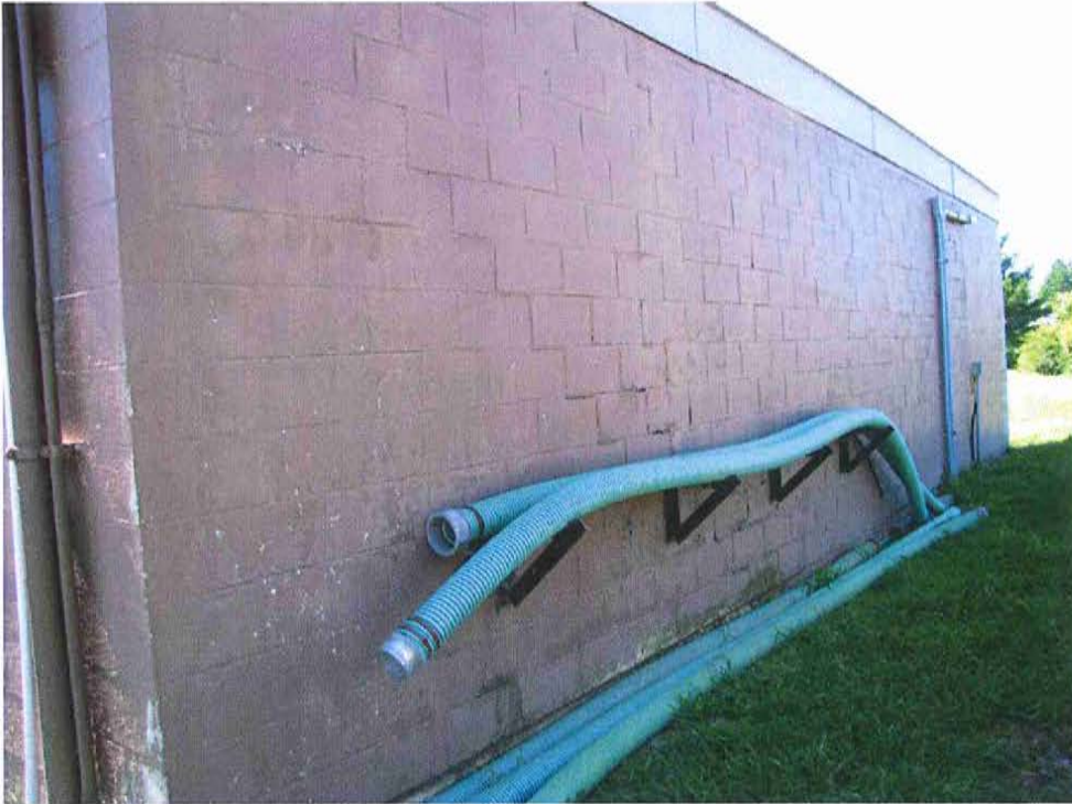
Photo 73: Intermediate Pump Station - View of north wall looking west, showing paint degradation and more moss growing in the mortar joints and on the wall face.
